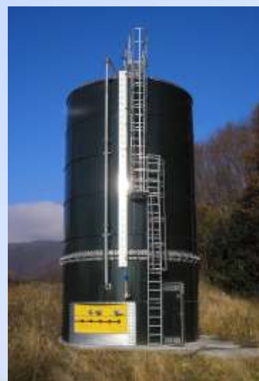
Silo Arona, Italy
